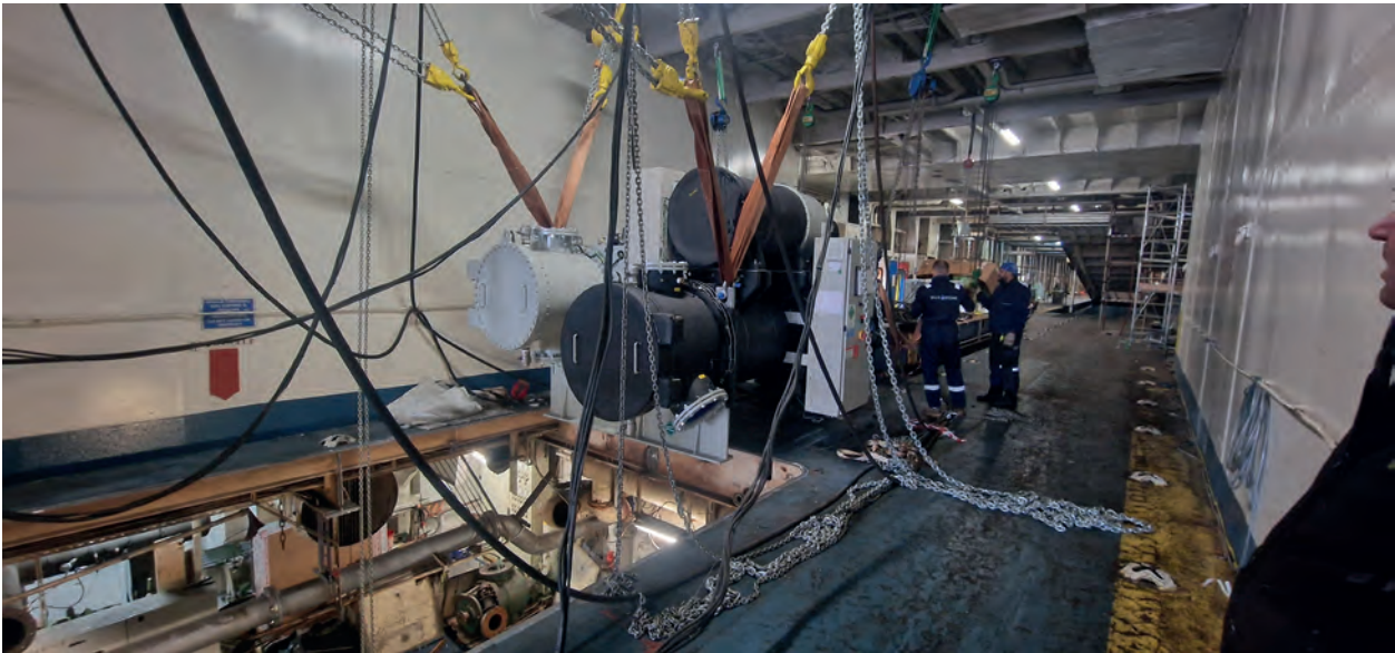
Bluestone workers rigging up a new high-efficiency chiller unit on a passenger vessel: the group has worked with many ferry and cruise operators
