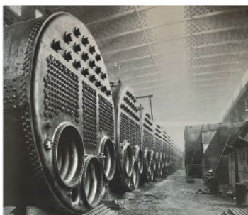
THE ENORMOUS DOUBLE-ENDED SCOTCH BOILERS DESTINED FOR BRITANNIC (1915) IN HARLAND & WOLFF'S BOILER SHOP
